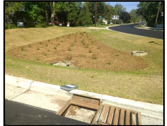
Structure located upstream of infiltration basin
